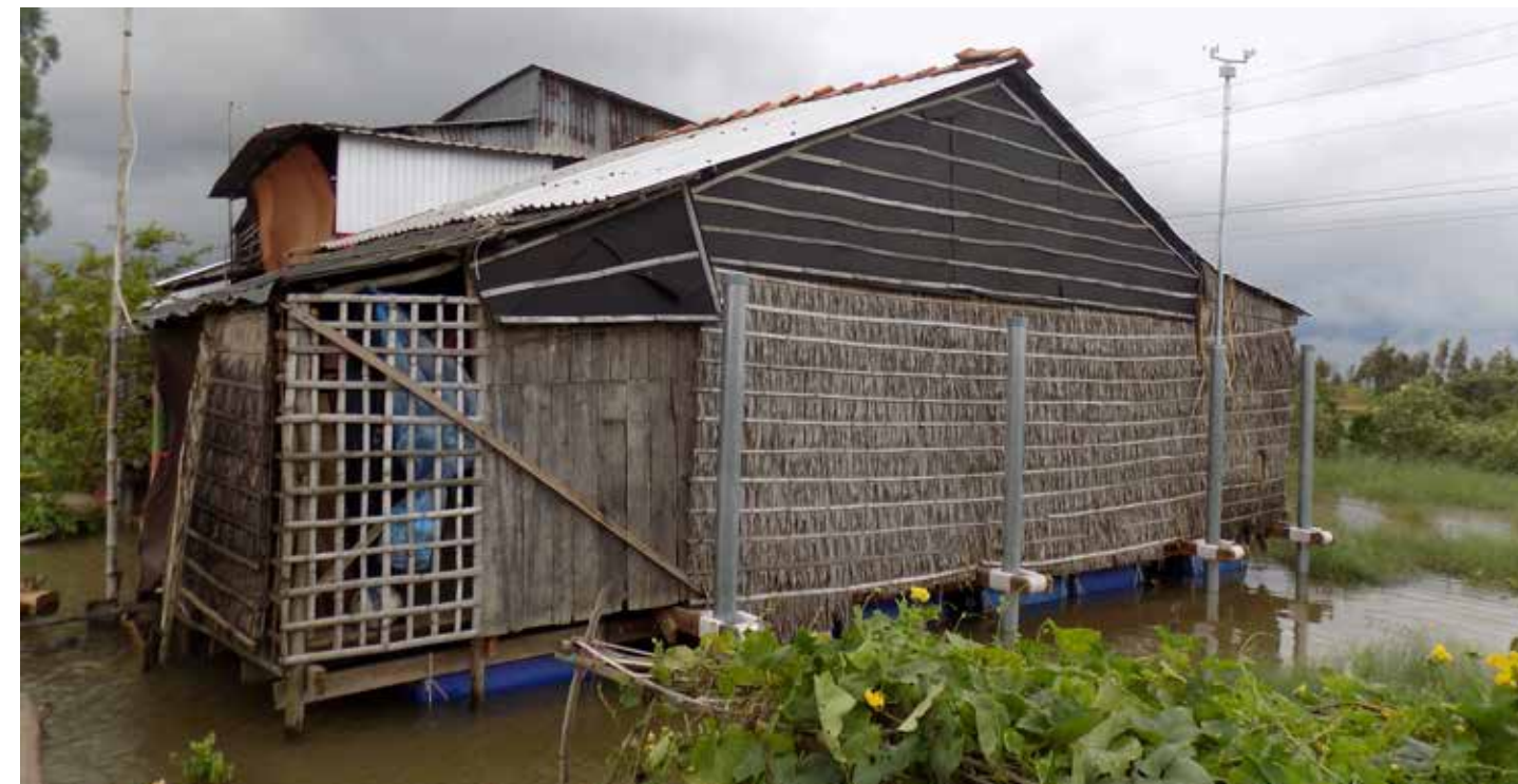
Amphibiated house floating on floodwater
