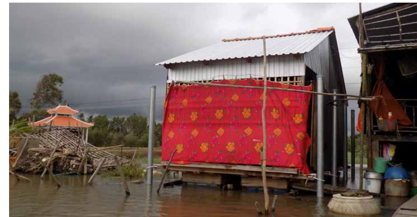
Amphibiated house floating on floodwater
